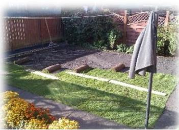
Turf being carefully laid, rolled-out, quite literally! – brick-like style to break the joints
